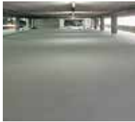
6. The surface is then finished with Triflex Cryl Finish 209.
