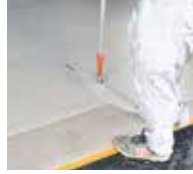
4. ... and spread evenly using a Triflex toothed rubber squeegee.
