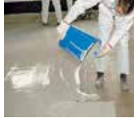
3. Triflex DeckFloor self-levelling mortar is applied ...
