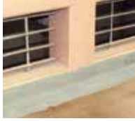
2. The details are waterproofed using Triflex ProDetail.
