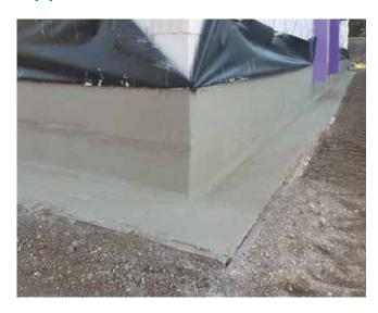
Waterproofing of the structure starts with the foundations being properly and professionally laid. The material used has to meet the challenges of a high water table and rainwater. Only reliable waterproofing of the foundation and base will ensure the durability of a building.
