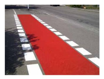
**Preco Cryl Roller-Applied Plastic 2K** is used as a textured and non-slip coating for surfaces and cycle paths, including those which run alongside the main flow of traffic. The completely elastic and non-slip surface cures in less than twenty minutes.
