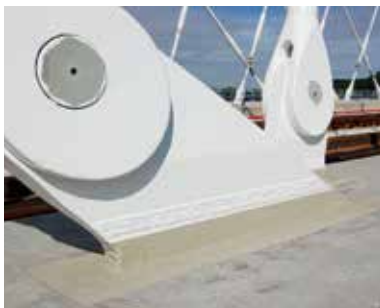
Troja Bridge, Prague (CZ)
